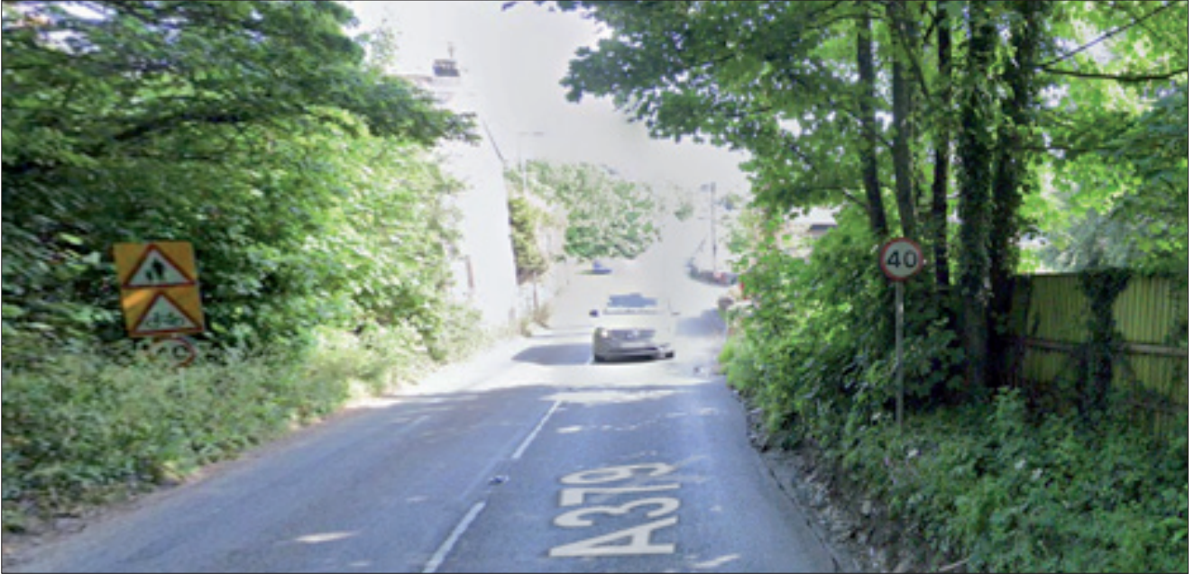
The road crossing at the bottom of Aveton Gifford hill is hazardous to reach the footpath.
