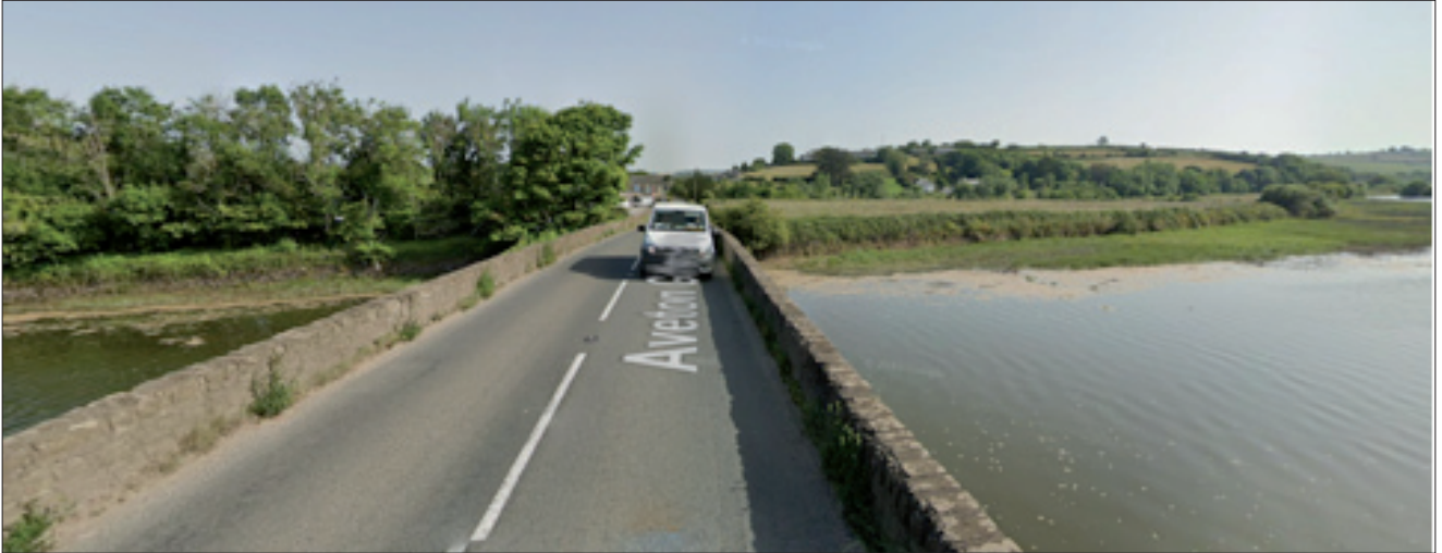
After entering the highway, the street lighting ends and the only escape route for a pedestrian is to jump over the wall, tide in or tide out.
