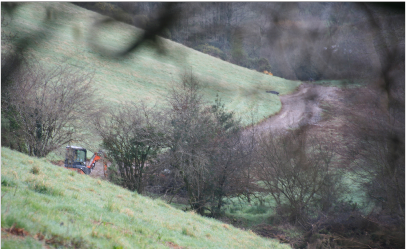
The steepness of the slope ensures it drains quickly and surfacings from the track could wash in to the stream to the right
