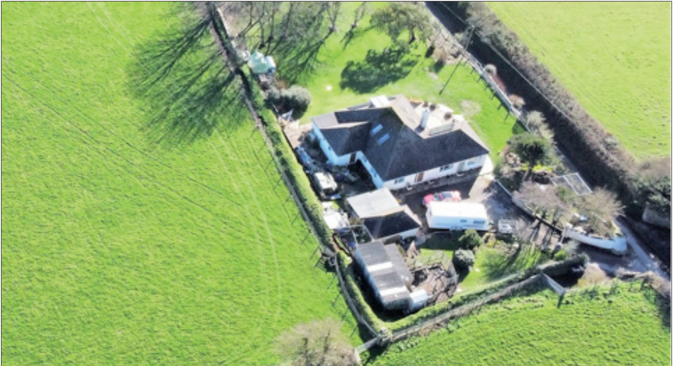
Higher Manor in 2021, before work on the site began
