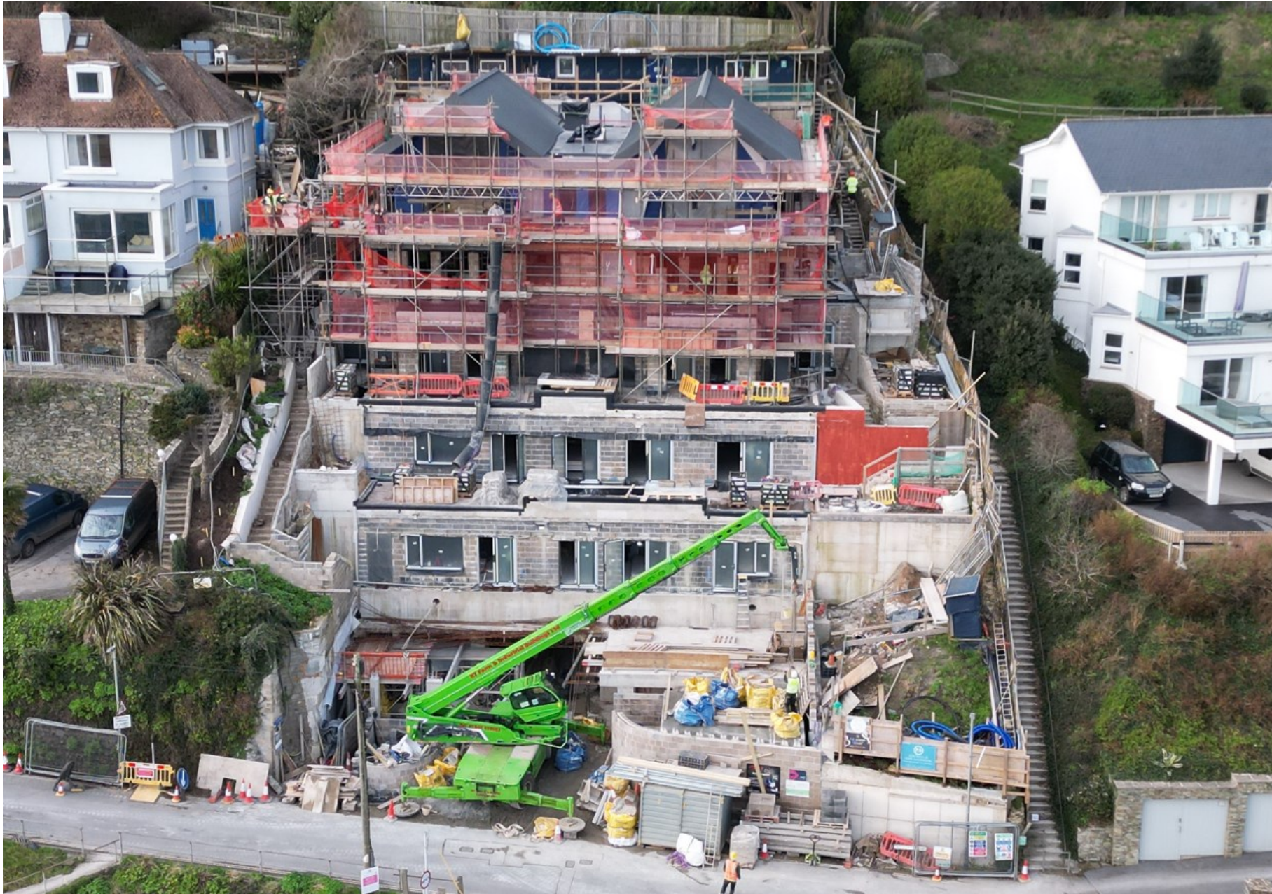
Boundary to boundary concrete Spion Lodge development.
