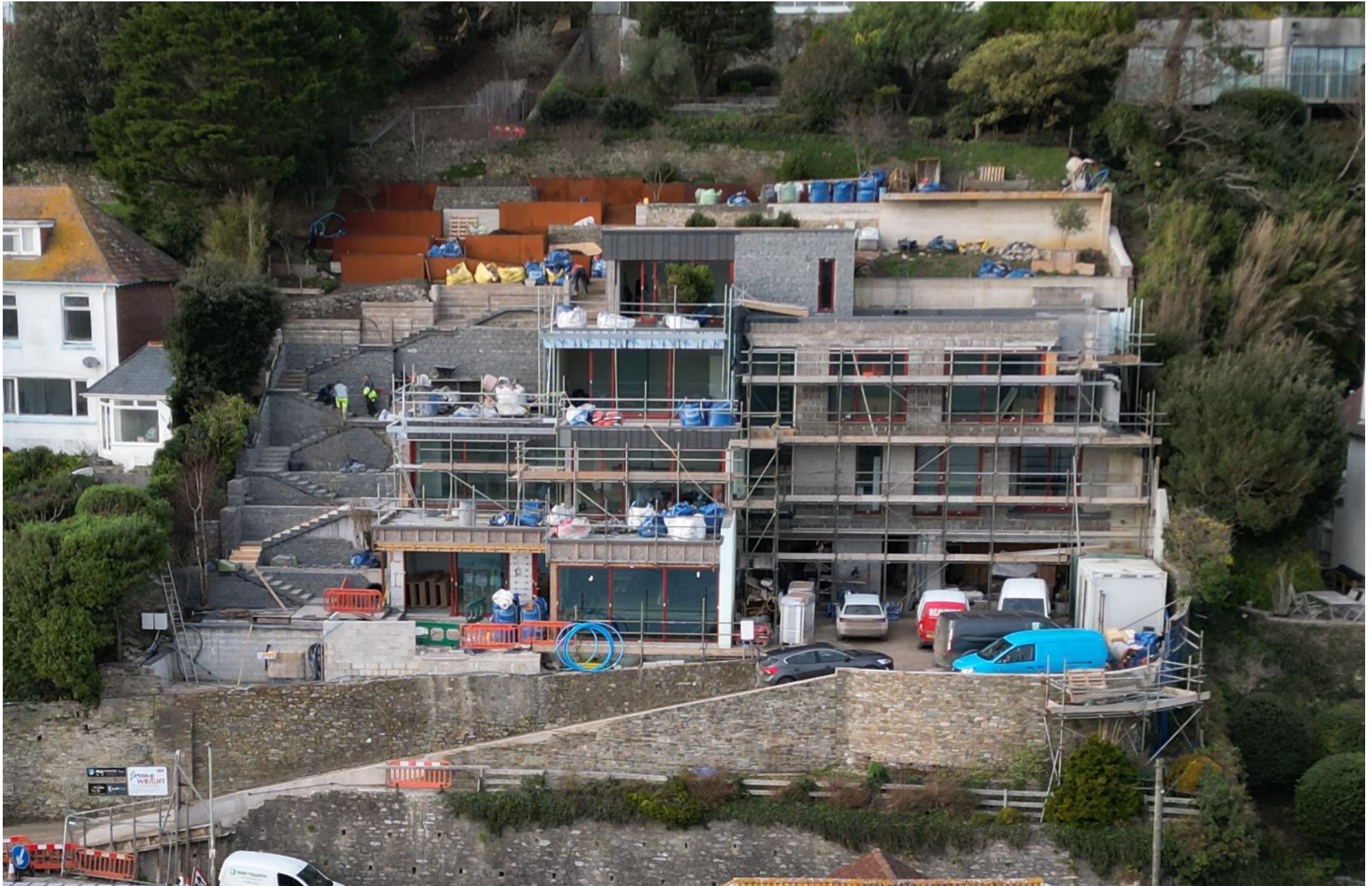
Boundary to boundary concrete Herwood development.
