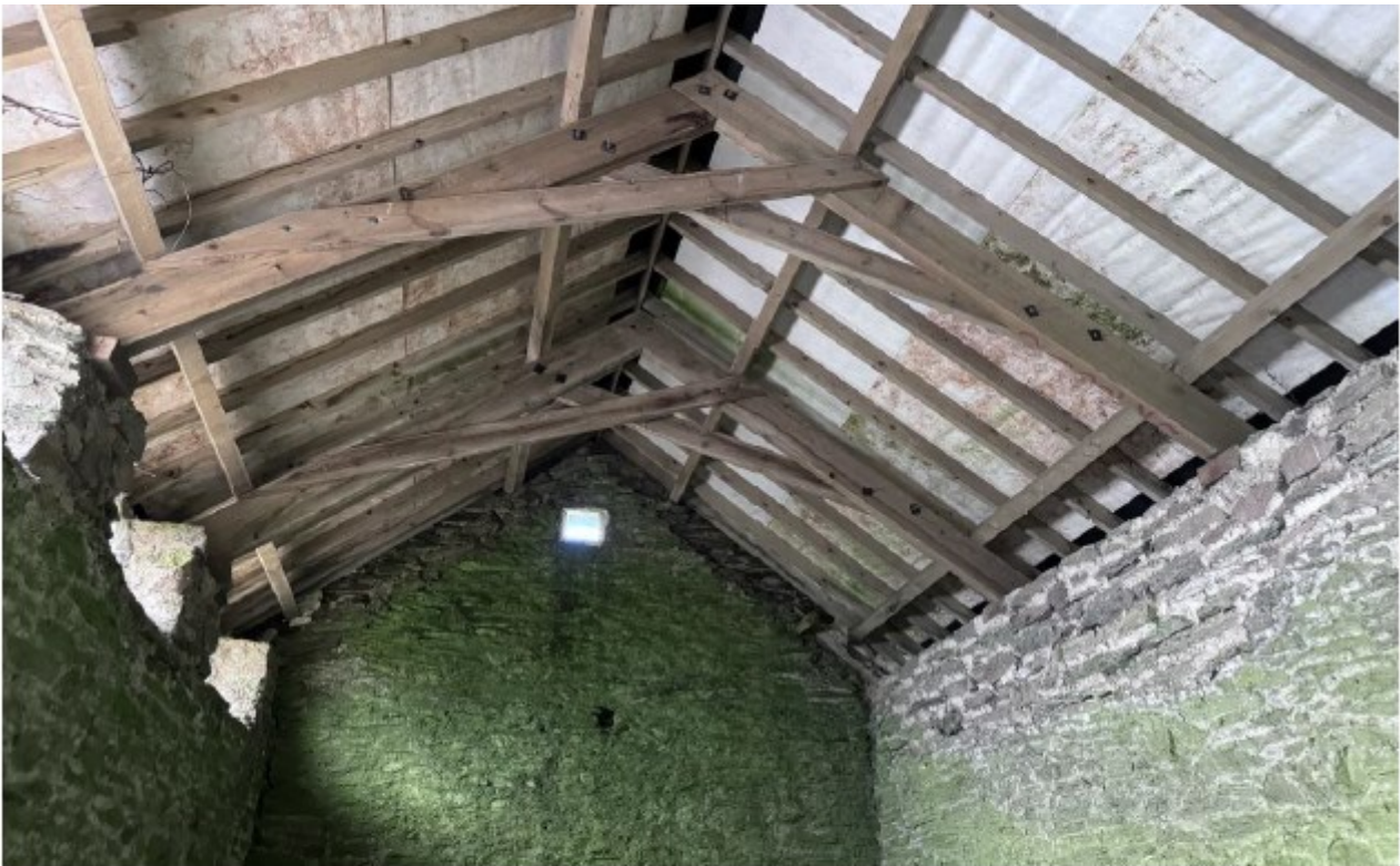
Figure 4 – Roof structure in good condition.
