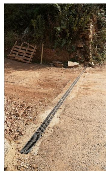
Where a stone wall once stood, a new drain channel has been installed:
