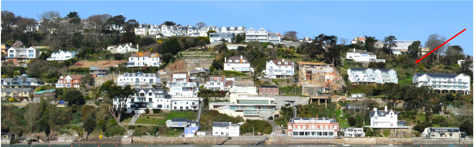
The hillside, is being ripped apart, plot by plot (above 2021- below 2024)
