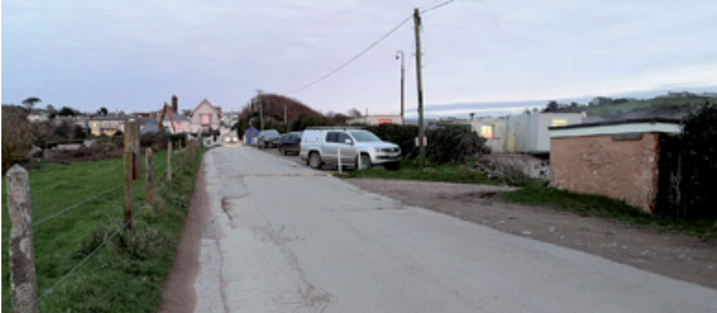
The construction compound that should have been removed remains visible to the right
