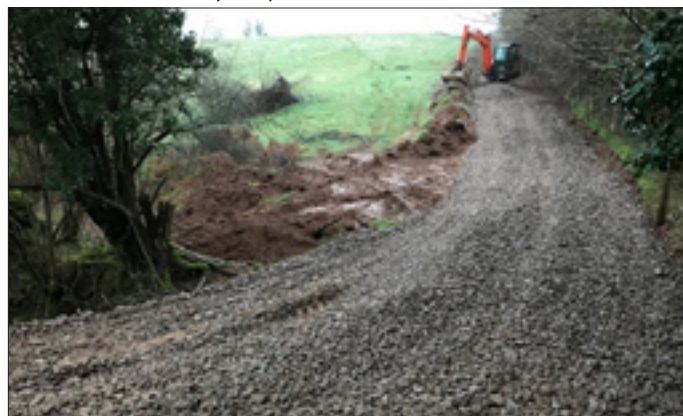
The track being constructed
