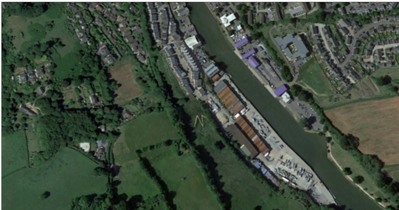
The Acorn Property Group and the TQ9 Partnership wish to replace many of the marine facilities with shops, restaurants and housing
