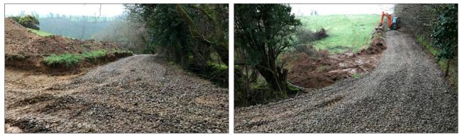
As the photographs above show the track has been constructed without planning permission to a minimum depth of 150mm and immediately adjacent to both trees and hedgerows.
