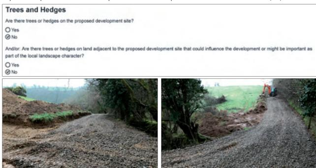
As the photographs above show the track has been constructed without planning permission to a minimum depth of 150mm and immediately adjacent to both trees and hedgerows.
